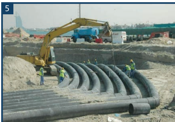
5 PE100 SDR11 10bar D630 Dubai Atlantis Project
