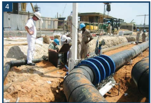
4 PE100 SDR11 10bar D630 Dubai Atlantis Project
